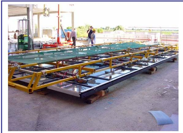
The special attachment of the glass-holding cleats of RP steel-glass facades to the carrying profile frame was made possible only through the use of special vacuum lifting technology from us, Germany because when such an element is lifted via the glass, this special attachment is the critical link in the chain.
