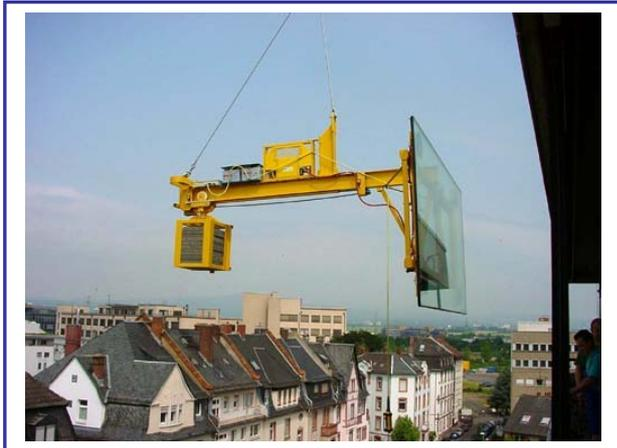
The company Normbau Weity GmbH & Co. KG of Ortenberg-Lißberg was faced with exactly that problem during the reconstruction of an office building in Frankfurt Rödelheim: Around 90 insulating glass panes were scheduled to be replaced by smaller window elements in the five-floor office building.
