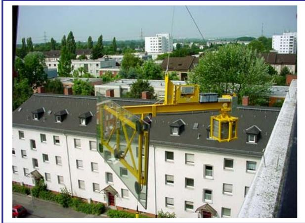
The vacuum generation was done using a separate battery-operated vacuum unit. Pannkoke's concept enabled a quick adjustment to the new operating conditions and a vacuum unit to be used for other cases. The modular structure of the device enabled a quick exchange/replacement of the vacuum unit. Thus, the device could be quickly converted if the construction supervisors demanded a redundant vacuum system.
