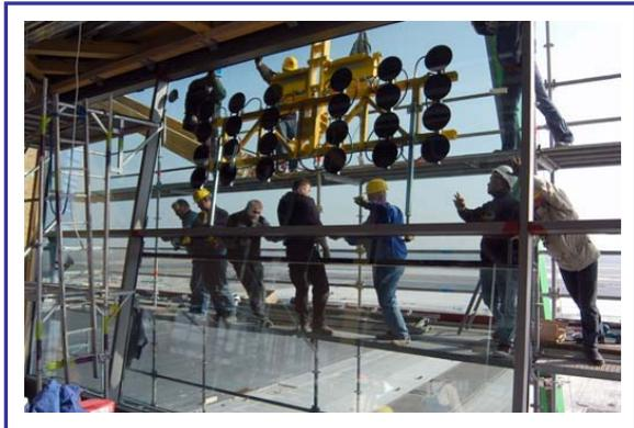
A giant mobile crane with a radio remote control supported the experienced staff of the Zange company as well as the vacuum lifting devices of us, enabling them to successfully execute the glazing at an inclination angle of 9°.
