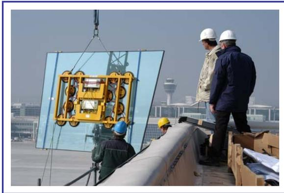
In addition to the vacuum lifting device Kombi 7211-CeDe for the large insulating glass panes, the smaller battery-operated vacuum lifting device Kombi 7211-VT from us was also used. This device is also designed with the 2-circuit technology.
