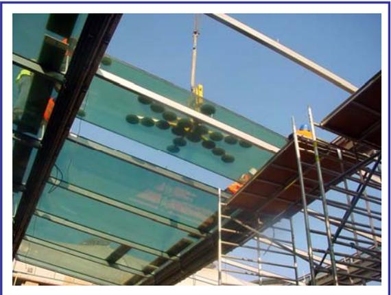
For the glazing to the roof of Dresden's main station and for other projects, Glas Zange extended the machinery required for such glazing work to include the **battery-powered vacuum lifting device KOMBI 7211-DS3**.
