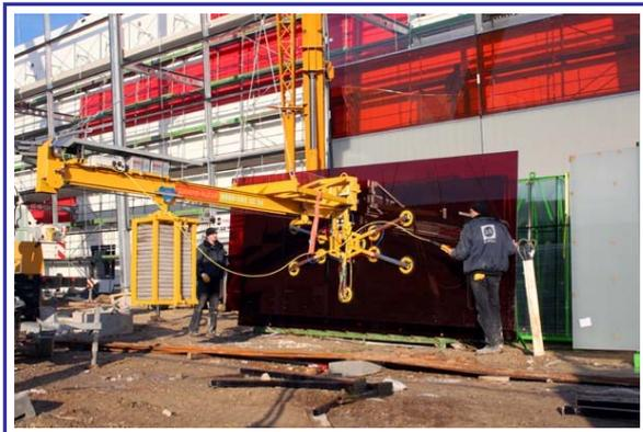
Kuball will use Pannhoke Flachglastechnik GmbH of Lübeck's know-how to select the right devices for the project. However, instead of a simple vacuum lifting device, the company wants a multi-use device for the task, such as the battery-operated vacuum lifting device Kombi 7211-DS3.
