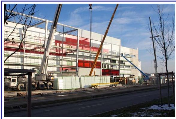
A major German furniture company has found a new look for its outlets! Including an extensive and colored overhead glass curtain wall. 5000m<sup>2</sup> colored laminated glass panes per construction object will be mounted into the steel curtain wall, that is tilted outward.
