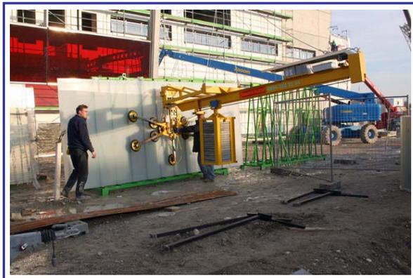
The combination with the counterweight unit Balance5 enables the vacuum lifting device to handle the outward-tilted steel curtain walling.
