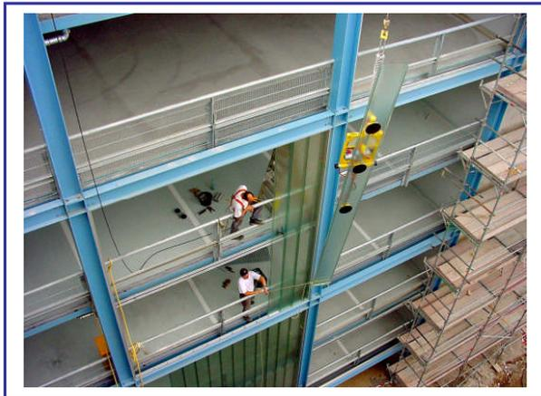
**For a parking garage construction in Frankfurt/Main, Germany at the exhibition area at Rebstockpark, Messrs Terlinden - transparent constructing - from Xanten, Germany received the order to install 10.000 m<sup>2</sup> Profilit Glass and this with a glass length of over 5,30 m.**
