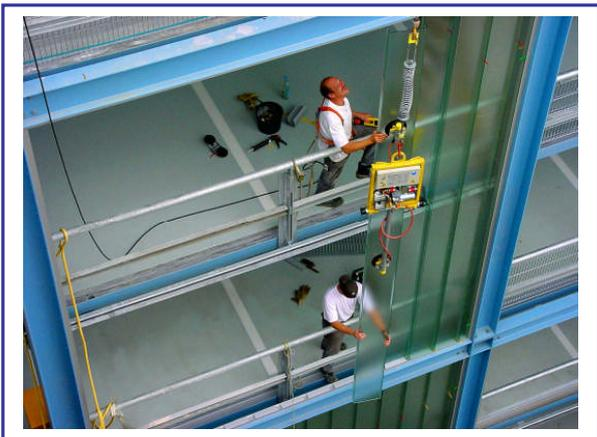
The company Terlinden came to us and explained their problem. Within a short period of time we got a special vacuum lifter with the suction cups arranged three on top of each other. The chosen mobile crane was equipped with two chain tensions in order to control the lifting movements quicker and more efficiently. With this device combination it was now possible to glaze economically and without a risk the over 5,30 m long Profilit Glass lines.
