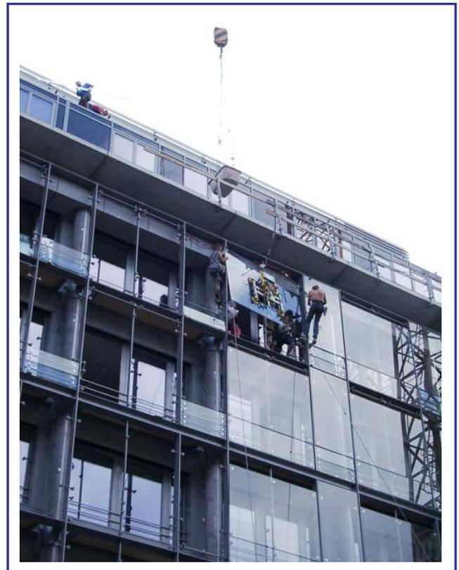
The photos were taken in July 2001 and show the setting of an approx. 300 kg glass pane under the projecting end of a roof - without a stage.
