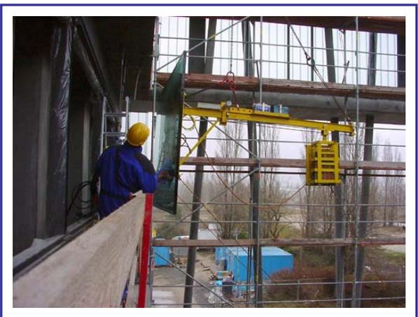
Bayer Glasbau GmbH from Berlin got the order to glaze the outer facade of a new building at the Humboldt University in Berlin with 7.000 m<sup>2</sup> of insulating glass. This at a height of up to 12 m with a sheet size of maximum 4 x 3 m and a weight of up to 800 kg.
