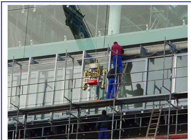
The company STEELWORK of Berlin received the order for the double glass facade of the new building, Deichtor Center, with a facade area of ca. 6,000 m<sup>2</sup>. This architecturally very interesting, three-sided and ca. 35 m high construction was designed by a Hamburg architectural firm, BRT.
