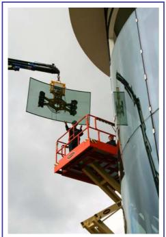
The "Montage van der Linde b.v." from Leimuiden, Netherlands ( www.montagevdlinde.nl ), specialist for difficult glazing applications, had the task of glazing a round arch for the Nieuwbouw Chinees Zakenhotel in Delft. Panel dimensions 2380 x 680 mm with a radius of 3900 mm to 2380 x 3740 mm and a radius of 4190 mm. maximum weight 490 kg.
