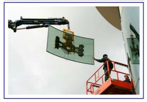
The curved special insulating glass panels for glazing came from the production of the "Franz Döring GmbH & Co. KG" Company from Berlin, Germany. "Franz Döring GmbH & Co. KG" also uses a multitude of various Pannkoke vacuum lifting devices in production.
